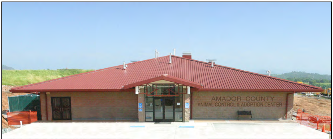
New Animal Control Building
