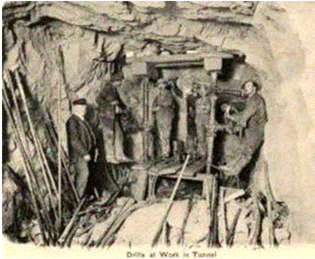
Miners at the hot and dirty work of drilling in the tunnels.
