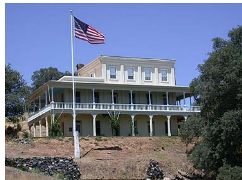
Kennedy Mine Office today.
