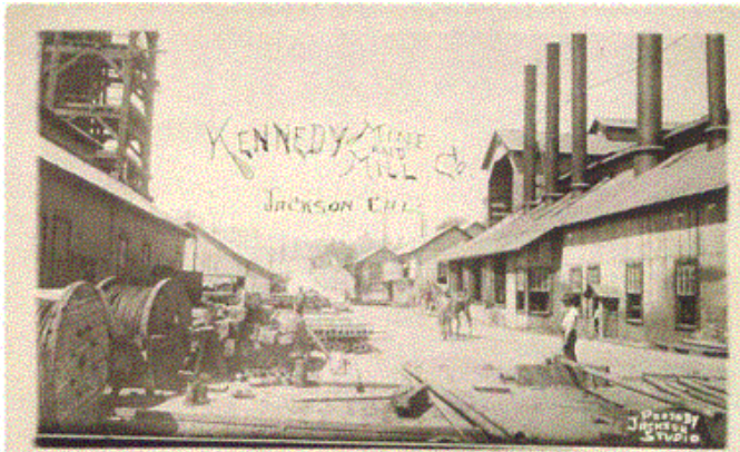
Older wood head frame and air intake stacks for the compressors.
